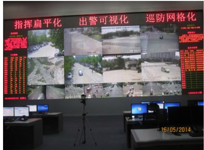
Command Centre in Weifang City
