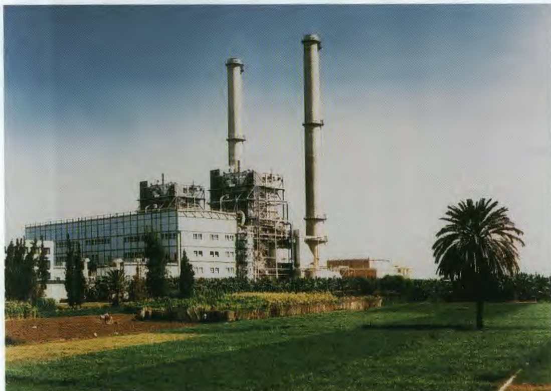
The Cairo West Power Station Extension Project, aimed at increasing electricity generation capacity, and using natural gas as a substitute for exportable oil and petroleum products.
