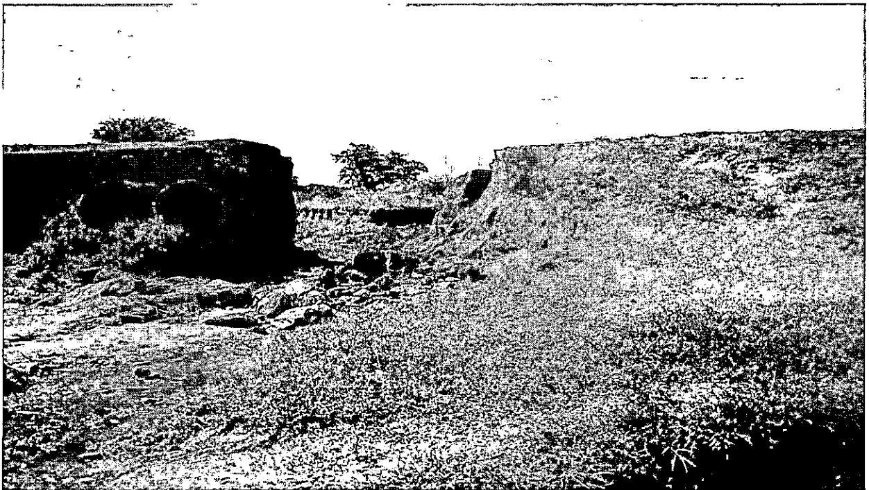
Collapsed bridge on the way to Talonna in northern Togo.
