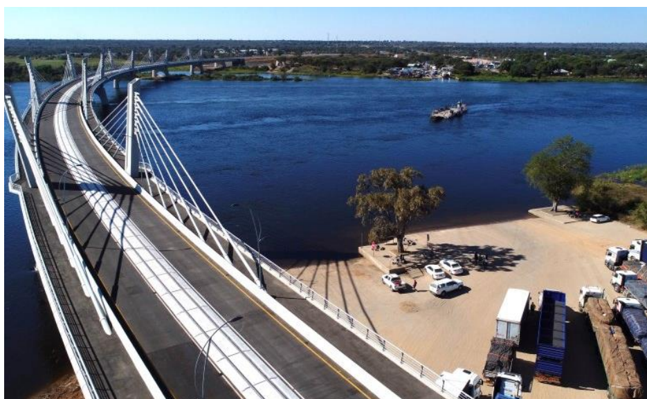
Photo: The Kazungula Bridge. Source: Ministry of Transport and Communications, Republic of Botswana
