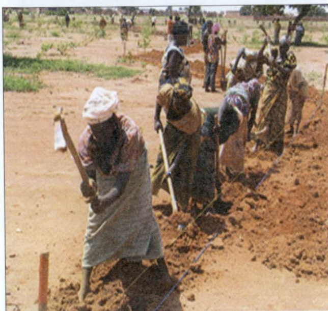
Photo 1 and 2: Building a rock bund using the PDS system in the northern area of Burkina Faso
