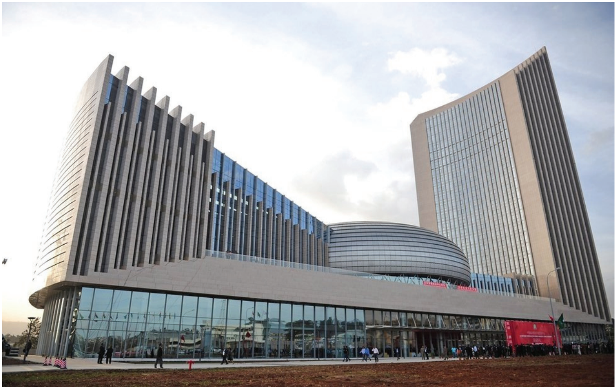
The new AU headquarters in Addis Ababa, Ethiopia
