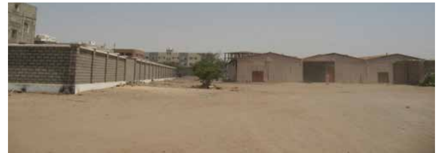
Figure 3 - This is the same ammunition store. It is in an unprotected light building with considerable urban development outside the compound, including one new apartment building within 100m.
