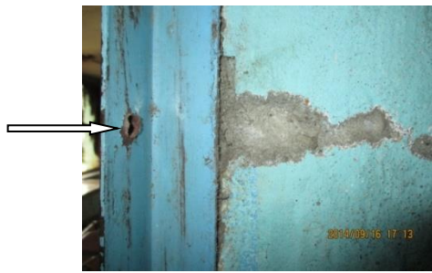
FIG 8: Door frame showing bullet mark 19 composed of a perforating defect through the metal of frame with inwardly-deflected metal edges and furrowed track across the adjacent paint/mortar or wall
